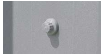
Correctly tightened colour-matched fastening.
