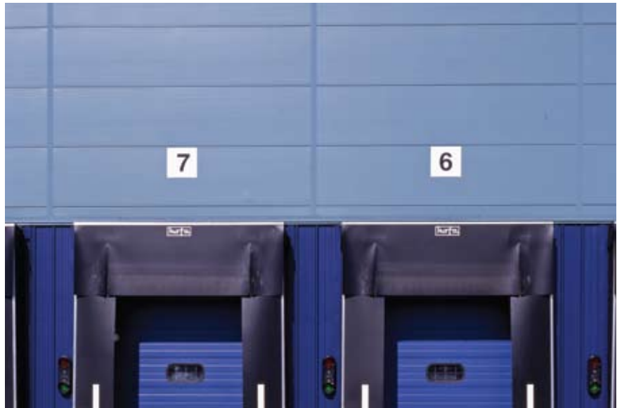
Vertical breaks incorporated into horizontal cladding.
