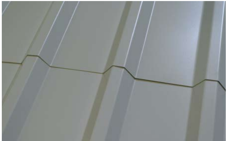
Tight overlap joint in accurately profiled sheets.
