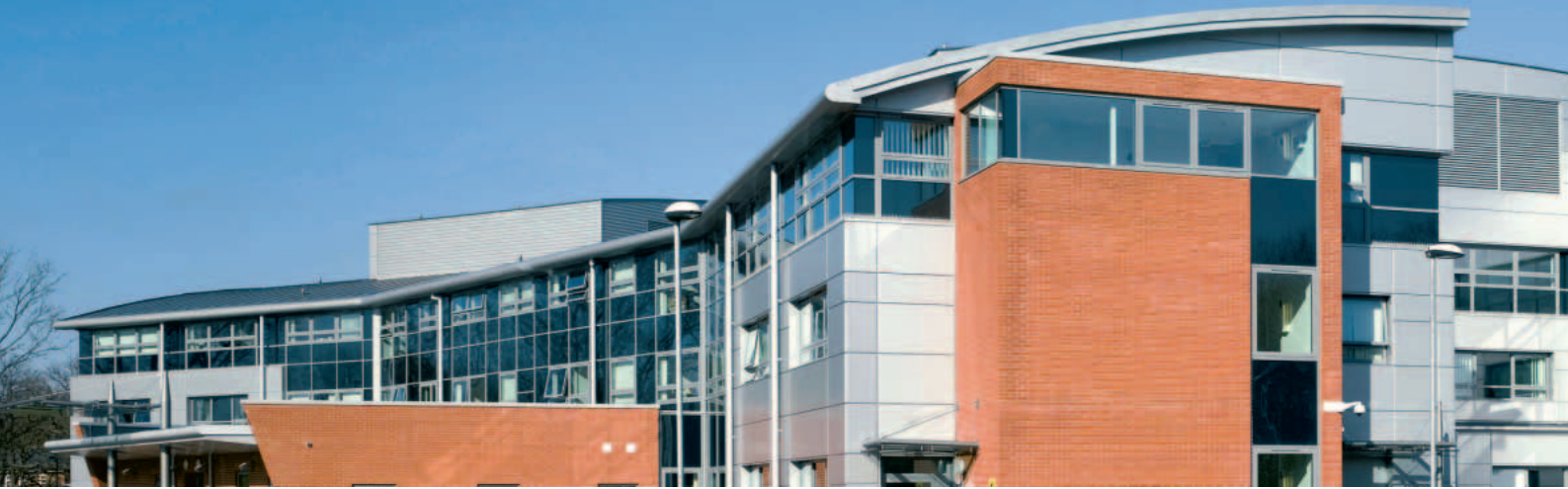
The Aldershot Centre for Health uses Colorcoat Prisma® pre-finished steel in Metallic Silver for the wall cladding.
