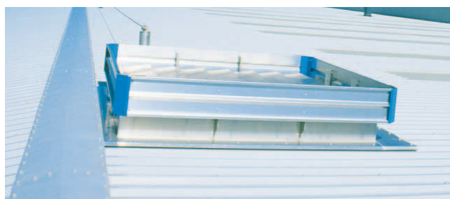
A penetration in roof cladding
